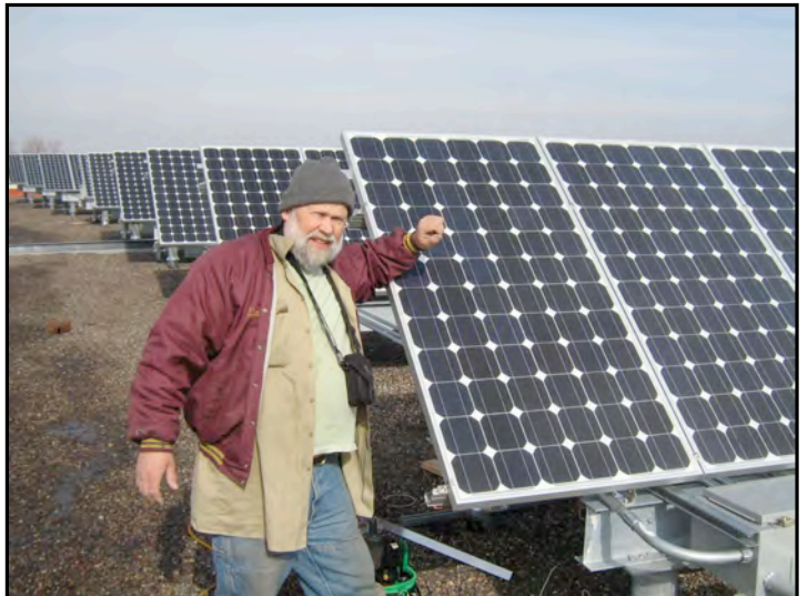
Figs. 11.-15. The Newly Installed PV Array on the Hennepin County Maintenance Center Roof in Medina is, at 98 kW capacity, now the largest PV system in Minnesota. The Wanxang cells were made in China.
