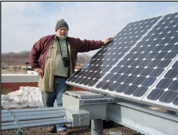
Figs. 11.-15. The Newly Installed PV Array on the Hennepin County Maintenance Center Roof in Medina is, at 98 kW capacity, now the largest PV system in Minnesota. The Wanxang cells were made in China.
